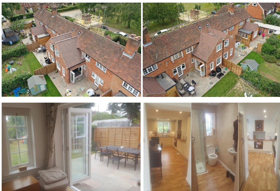
Above: Interior & aerial images of the extensions to Group F terrace
